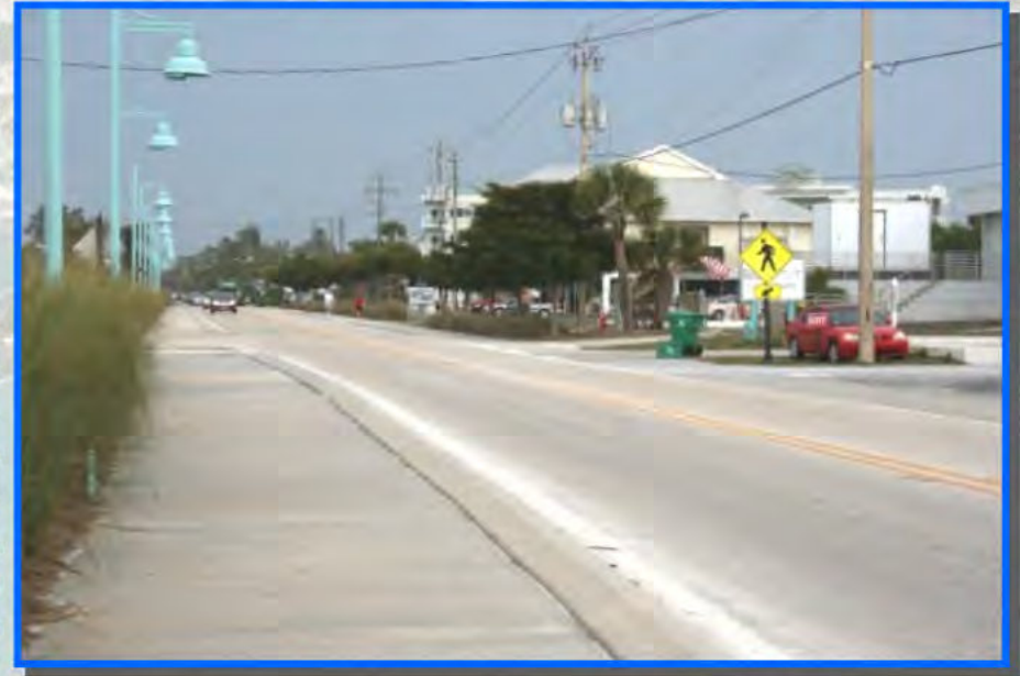
An 18 inch curb was constructed to separate the sidewalk from the travel lanes because they are on the same grade. This creates a dangerous conflict for bicyclists trying to utilize the street.
