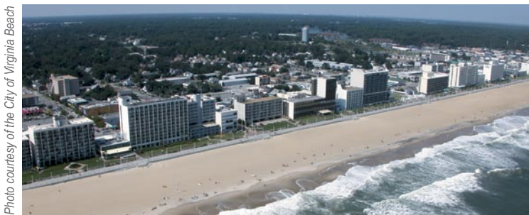
An estimated $105 million in damage was prevented after Hurricane Isabel struck a nourished beach with a seawall at Virginia Beach in fall 2003. 7 The project was designed to stop a 9-foot storm surge – and it did. The nourished beach minimized wave attack and overtopping of the seawall, the community’s last line of defense.
