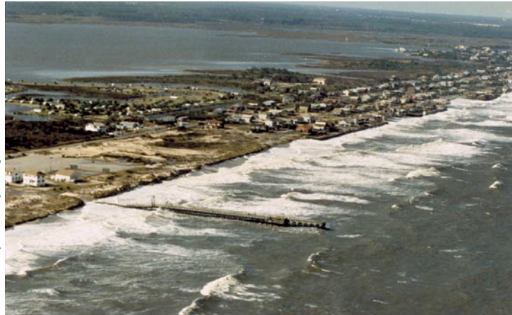
Storm waves break farther up on an eroding beach in 1991 at Sandbridge, Va., threatening people and property.
